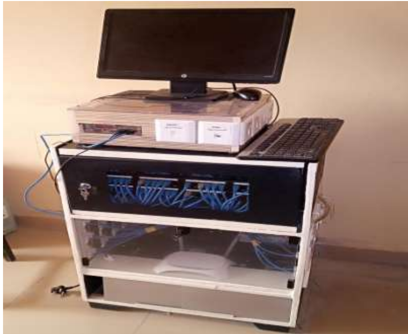
Figure 3: Complete View of the Fabrication
